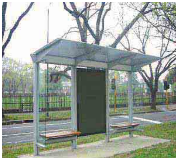
Bus Shelter with no advertisement panel
