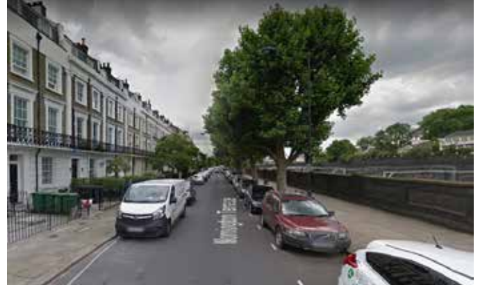
② A consistent domestic scale and form of buildings along Mornington Terrace is disrupted by an abrupt change in character with the rail cutting
