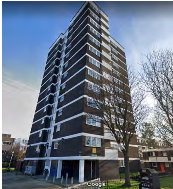
Image 2.4: Point block building (credit: Google)
