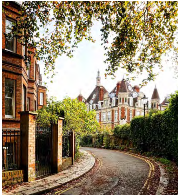
Image 2.1: Historic hospital building (Mt. Vernon)
