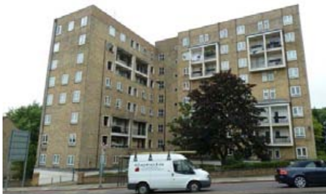
Substantial blocks in Swiss Cottage
