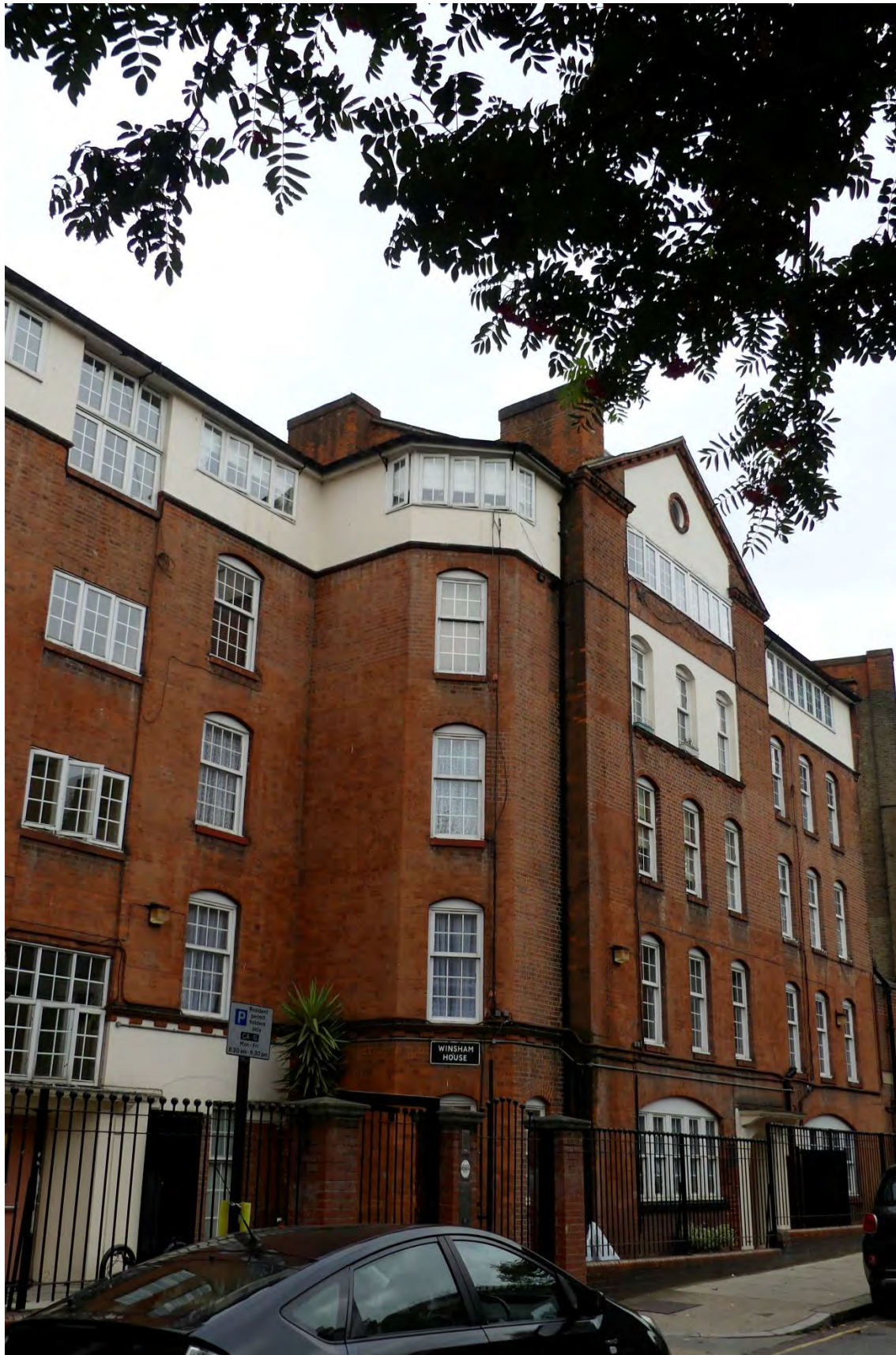
6.6.1 Churchway LCC buildings Winsham House. Photo RS.
