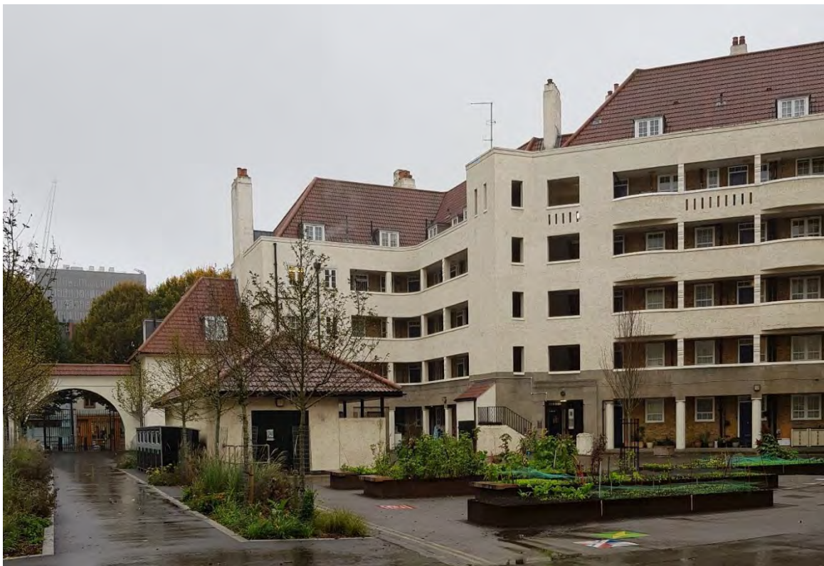
7.7.1 Ossulston estate, Levita House LCC. Photo RS.
