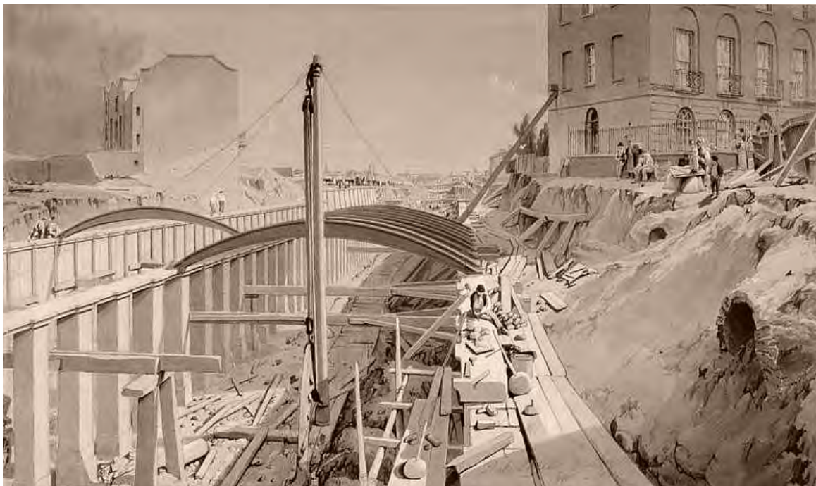
4.6 'The London & Birmingham Railway incline under Park Street, Camden Town, 18th September 1836', by J. C. Bourne (1837), tunnel building, looking south, under construction, with Stanhope Terrace to the right.
