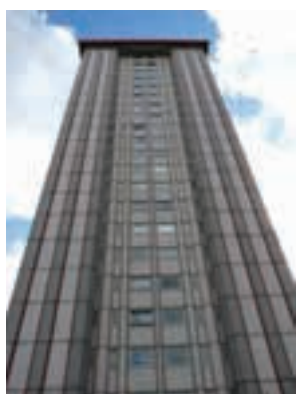
Amphill Estate towers
