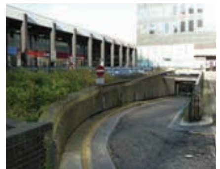
Free movement is impeded by service ramps.
