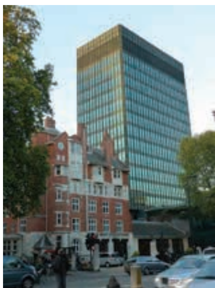
LCC fire station (1902) and Evergreen House.
