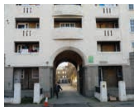
Entrance portal from Ossulston Street.
