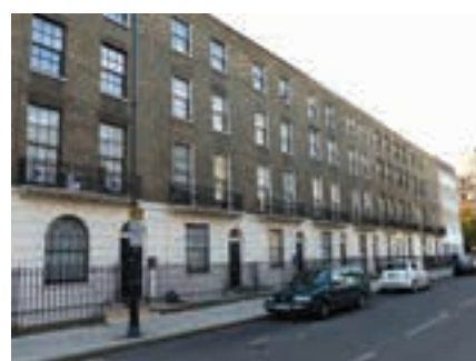
Four storey Georgian terrace, North Gower Street.
